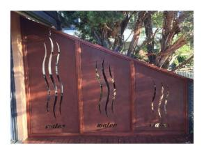
The image below shows an example of a screen half way through its sealing process.
