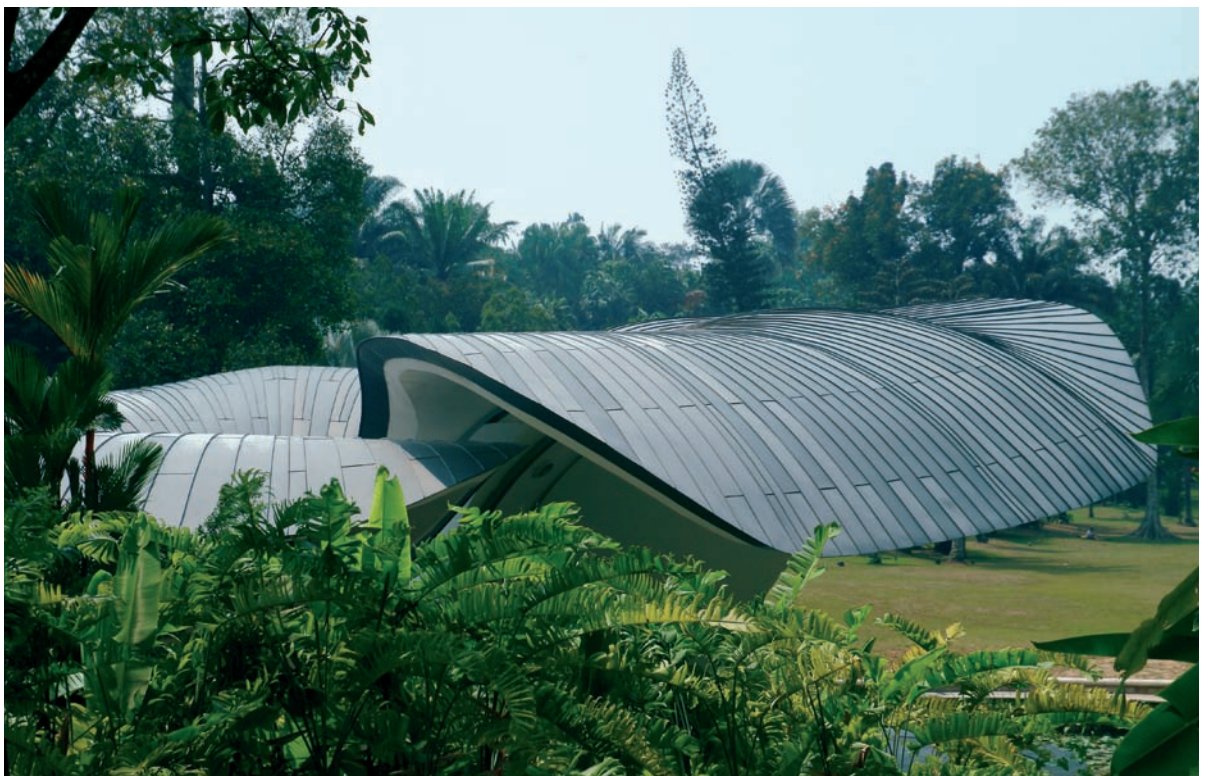
Auditorium symphonique Fondation Shaw (Singapore) - Architect: CPG Consultants
